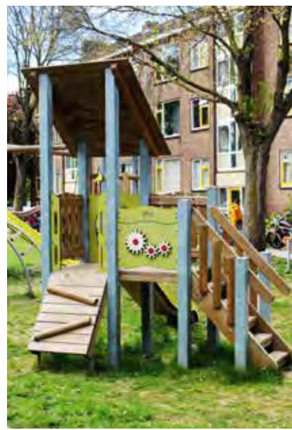
Images show unit with steel hot-dip galvanised posts
